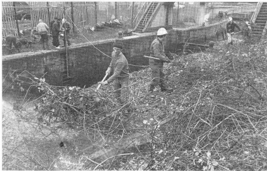
Clearance work at Carpenter's Road Lock, 2-3 March 1991
